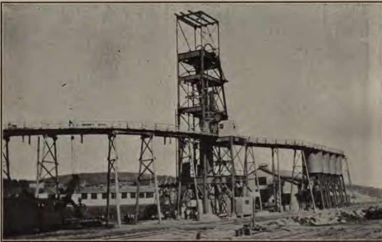
Brier Hill Mine, Penn Iron Mining Co., Vulcan, Mich. Steel Head Frame, Trestles and Circular Ore Pockets.
